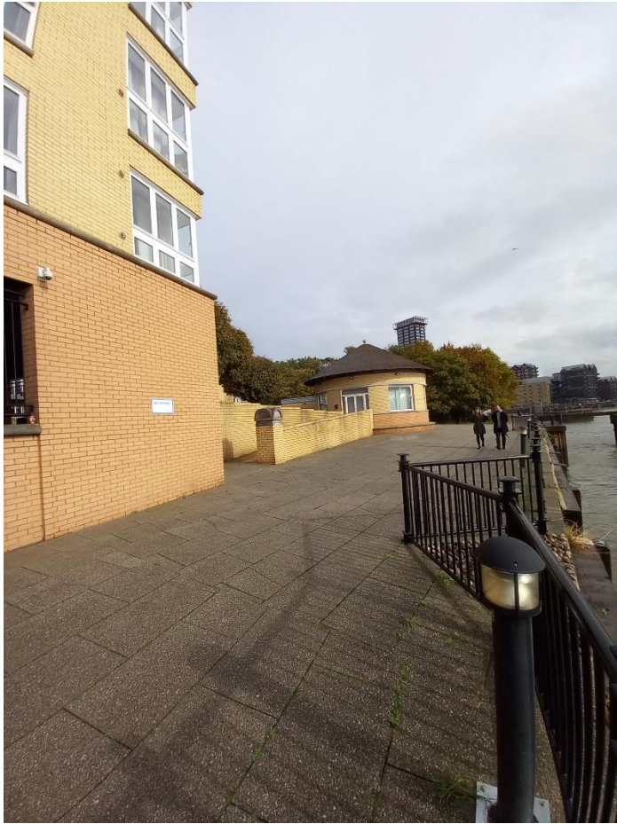
Image 7: Rotunda building and Thames pathway looking east
